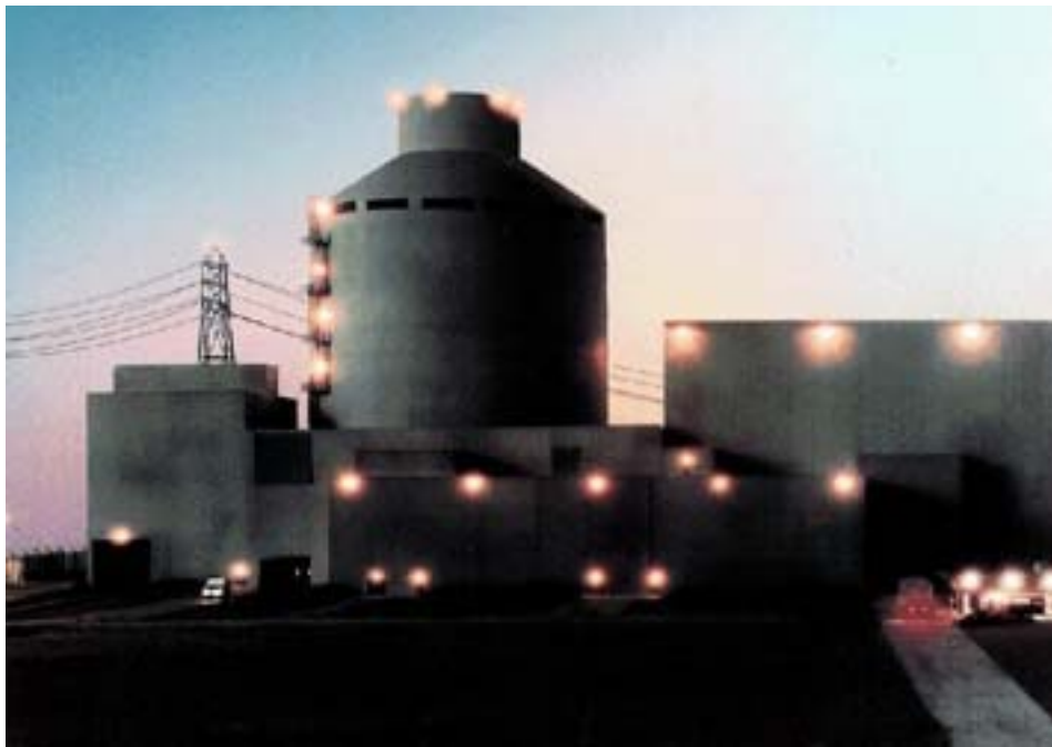
Figure 7. Advanced Passive AP1000 PWR includes a cooling chimney using natural convection in its containment structure.
